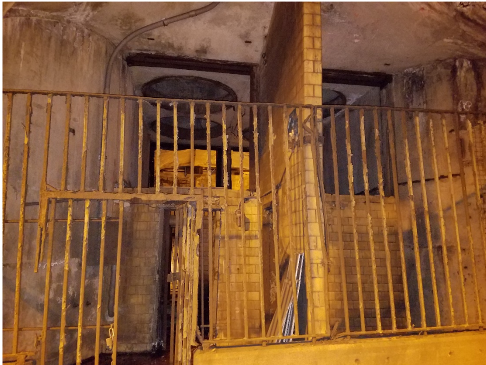
Photo 6: Gate entrance to abandoned control room.
