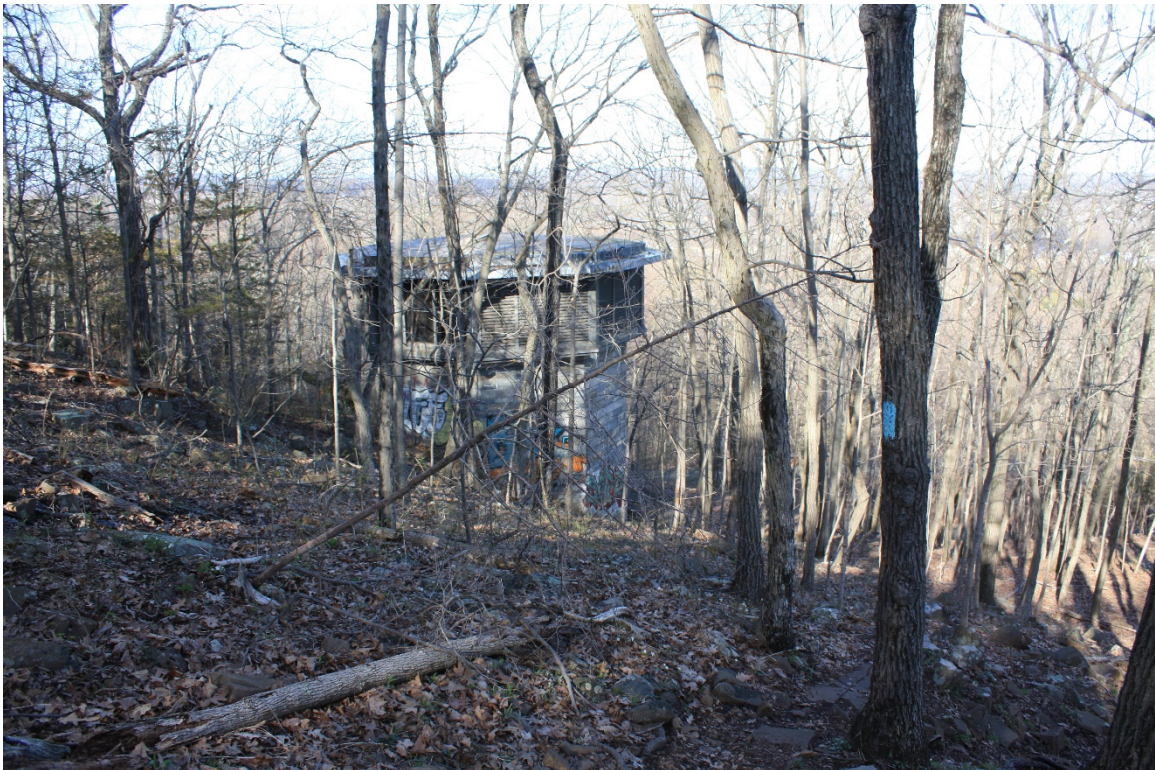
Photo 22: Ventilation Exhaust Building at top of West Rock Ridge.
