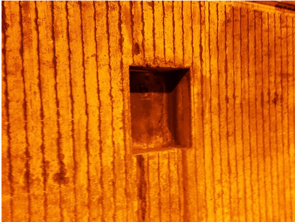
Photo 1: Remains of Ventilation Control Niche. Control System has been removed.
