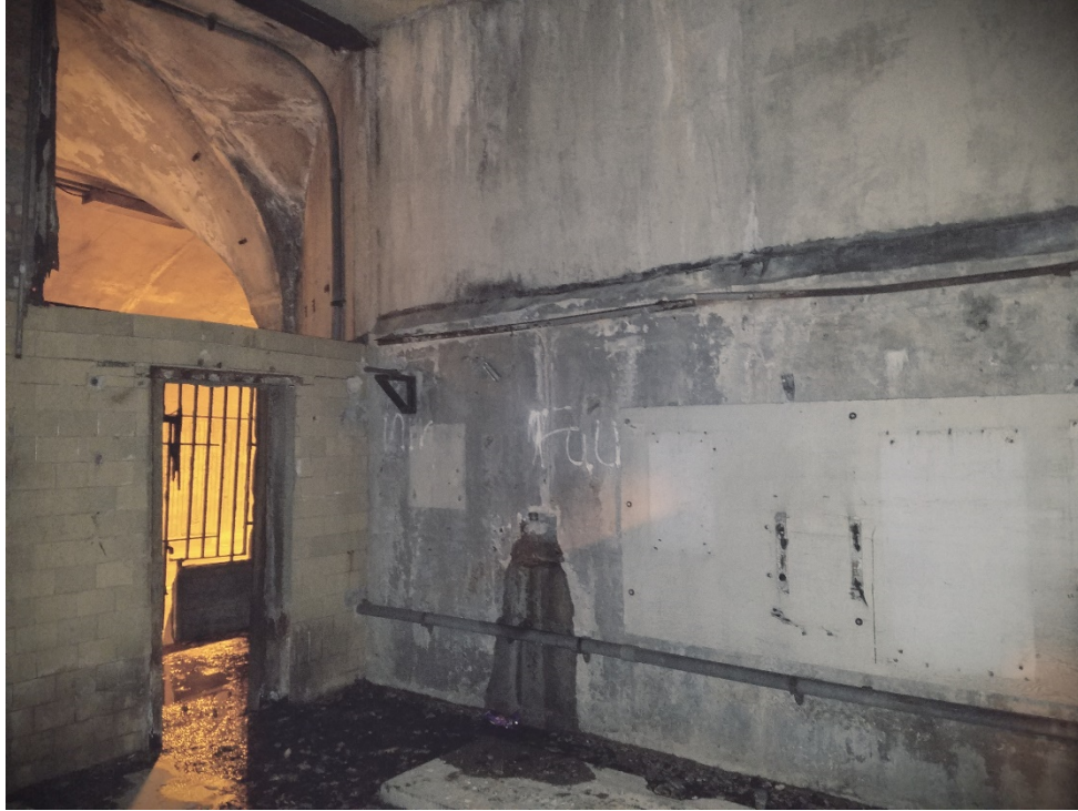
Photo 7: Interior of abandoned control room.
