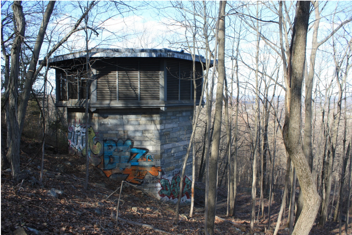
Photo 21: Ventilation Exhaust Building at top of West Rock Ridge.
